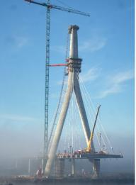
composite deck and the simultaneous installation and stressing of the cables.
